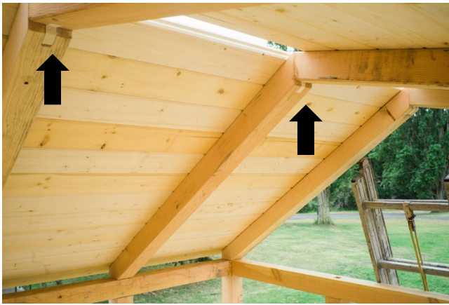
Figure 3. Roofing joinery takes the grain’s movement into account, while the small splines in the uppermost joints make for visually interesting wear as the wood moves and ages.
