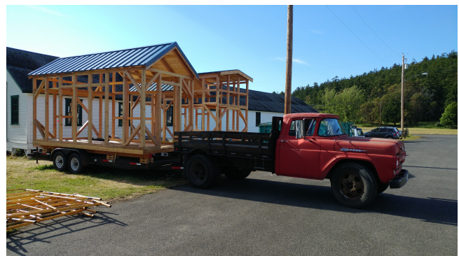
Figure 1. Completed tiny house frames being moved to their (semi)permanent sites
